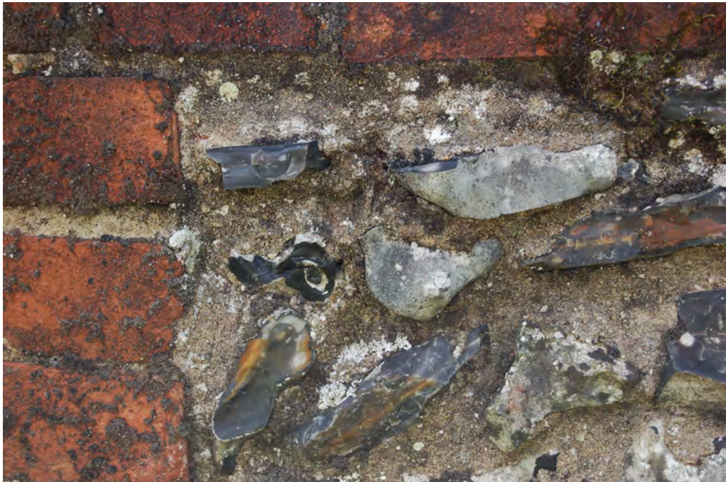
Picture 1.6 Traditional Essex flint panelling on the wall that defines the boundary of Pond Cottage.
